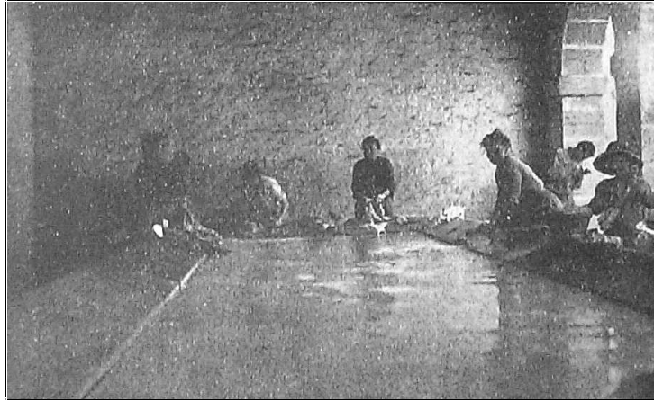
Public Washing Place – France, Chalindry
