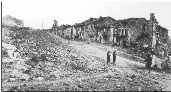
Signal Corps men stringing wires in Malancourt, October, 1918.
