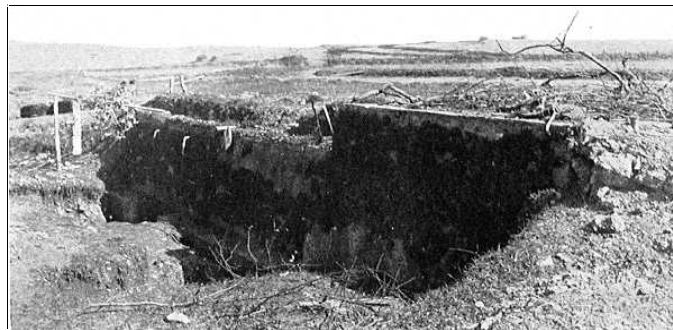
One of the concrete machine gun emplacements which were a part of the defenses of the Hindenburg line west of Preny. Similar emplacements were constructed at intervals of about 100 meters along the Tranche des Grognons behind the camouflaged road running west from Preny.
