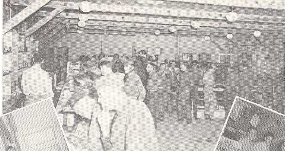
INTERIOR MAIN CAMP EXCHANGE
